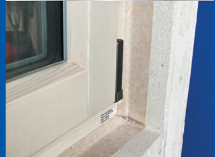
Window strip installation
